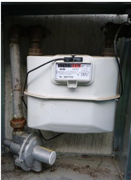
Contor gaz G6 debit max. 10 m 3 /h Generator impulsuri
