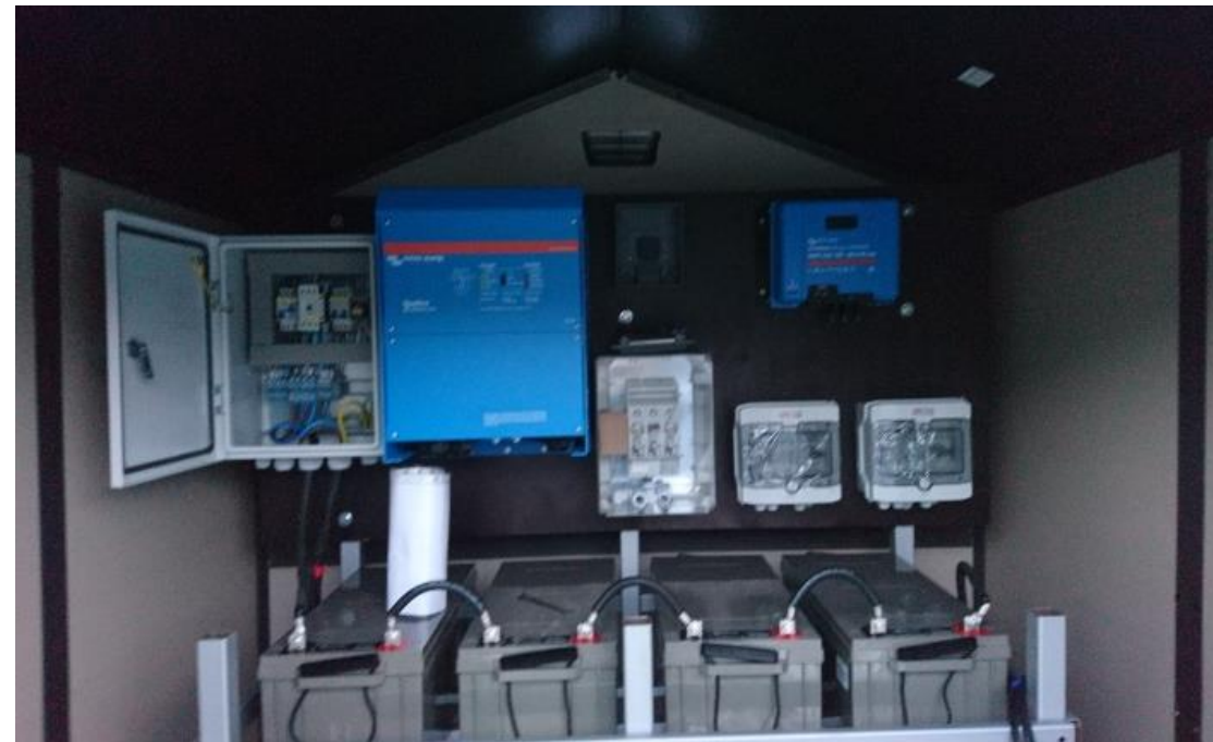
invertor off-grid 8 kW monofazat 12 acumulatori 12V, 220Ah
