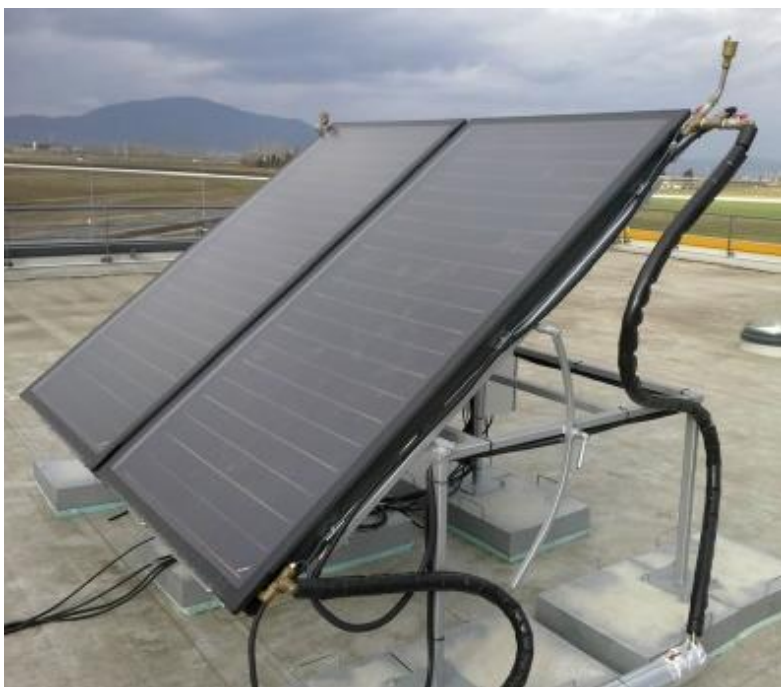
Colectoare solar termice plan plate S_a=2 \times 2,1 \text{ m}^2
