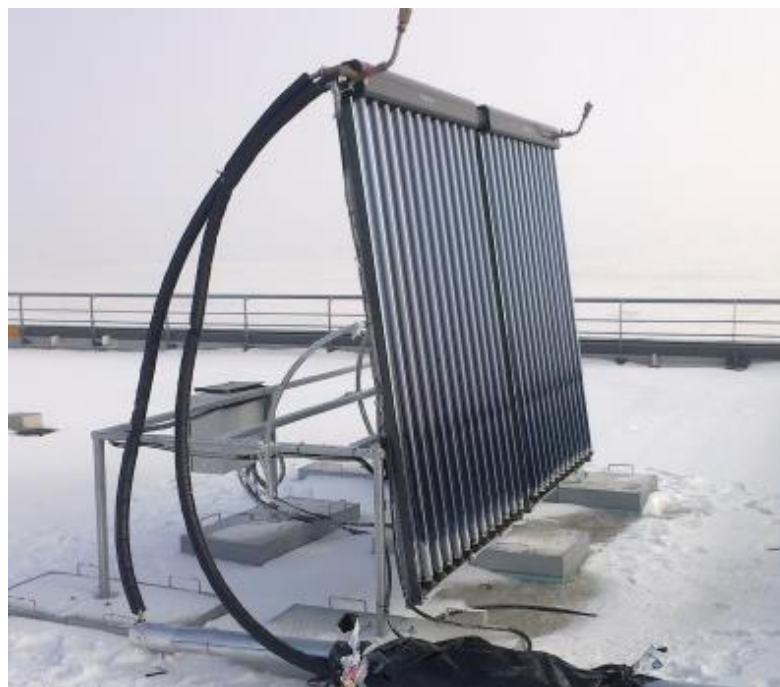
Colectoare solar termice tuburi vidate S_a=2 \times 2,58 \text{ m}^2
