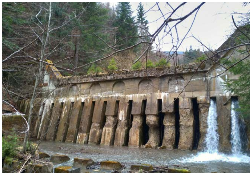
Fig. 5.33. Structure 10 BF 5,0 – Tigăi Valley, affected by erosion at the body structure level
