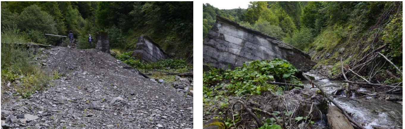
Fig. 5.22. Structure 90 BCF 2.0 - Vinderel Creek
