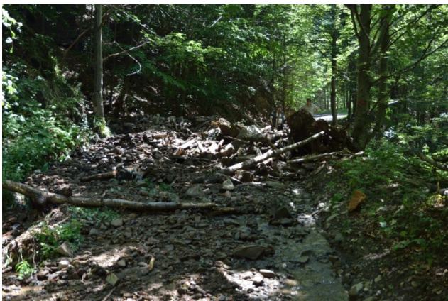
Fig. 1.1. Torrential transport plug on the forest road following the blocking of an evacuation bridge
