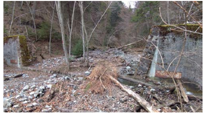
Fig. 5.9. Water course deviation due to apron silting (Mihalache, 2019)
